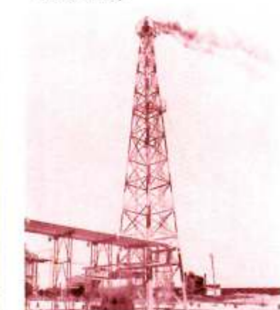
9 Flare Stack Plastic Resins & Chemicals
