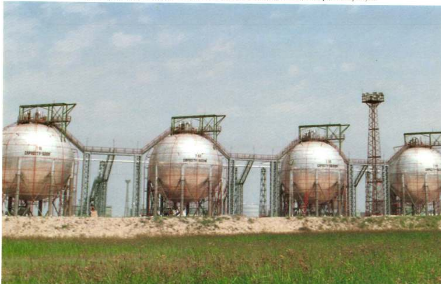
An EPC project for a LPG storage terminal consisting of 7 spheres handled for IOC's Panipat Refinery Project.
