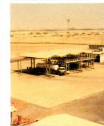
11 LPG Boiling Plant & Loading Gantry Brega Libya
