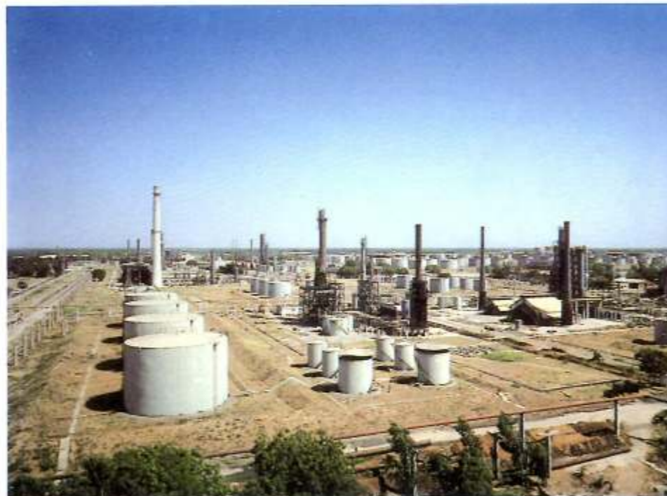
A diversified industrial project wherein VTV supplied a wide range of storage tanks, process column heat exchangers, gasholders and flare stacks.
