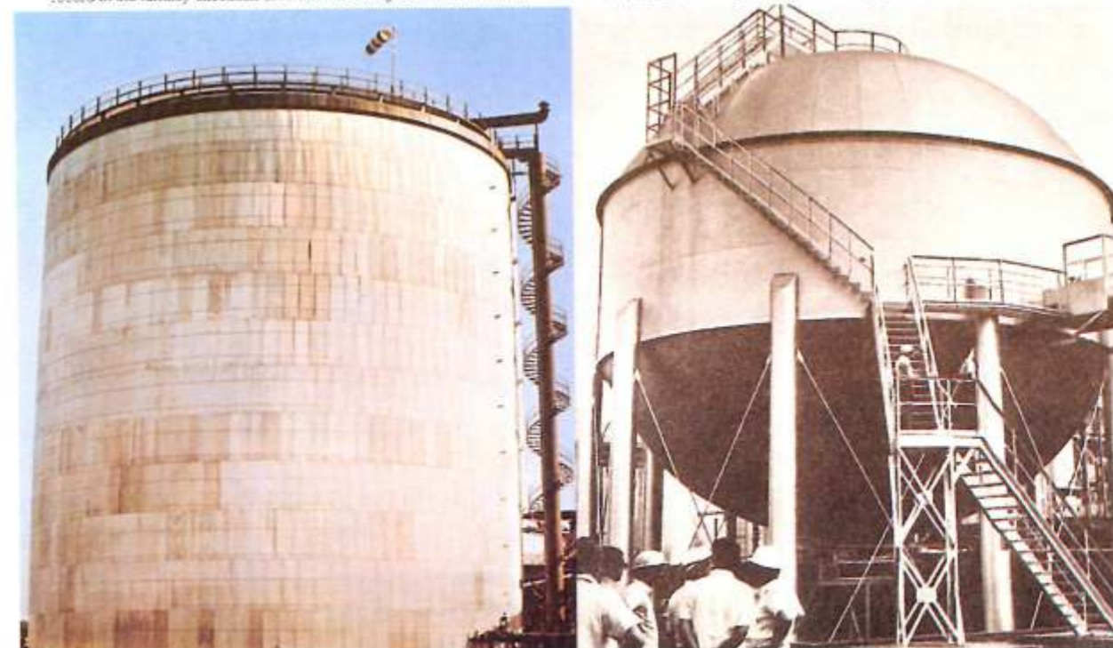
A 15000 cu.m. single wall insulated ammonia storage tank designed and constructed by VTV for GNFC, Bharuch. The dome roof was constructed at grade level and air raised to its final height. VTV has a very strong experience record in the turnkey execution of Ammonia Storage Terminals in India.
