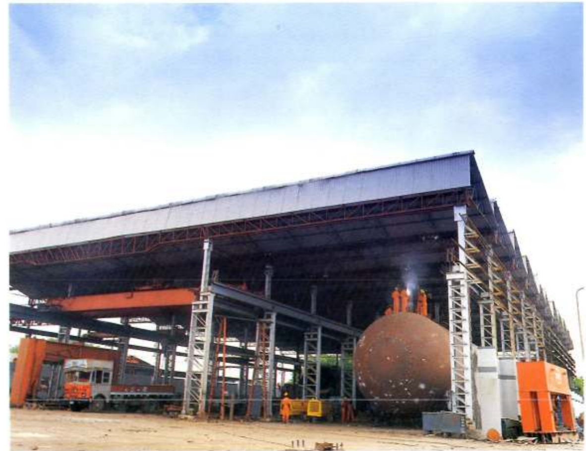
A 5.9 m diameter LPG bullet under final stages of fabrication at VTV's Baroda Pressure Vessel Factory. VTV's plants are designed to handle a multiplicity of overdimensioned vessels.
