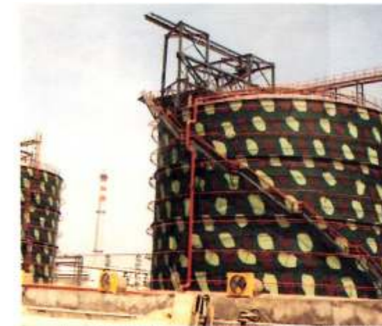
2 nos. 9% Nickel cryogenic double integrity ethylene tanks constructed for GAIL's Pata Petrochemical Complex.
