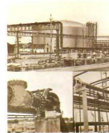
1 Cryogenic Ammonia Import Terminal Tutuohi
