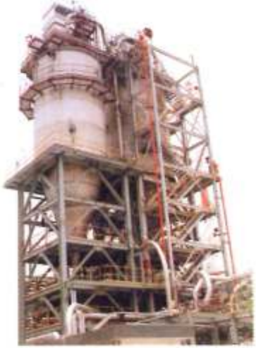
A silo designed and constructed for BIL's PTA plant at Hazira.
