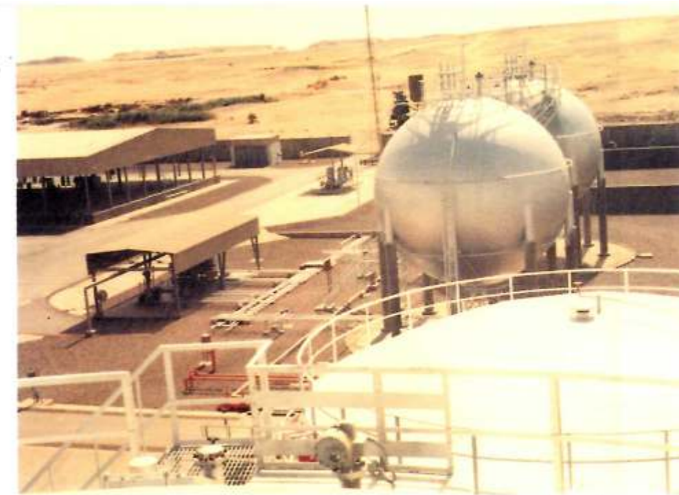
A US$ 33 million Petroleum & Gas Installation handled by VTV on an EPC basis in Libya, involving complete terminal facilities.
