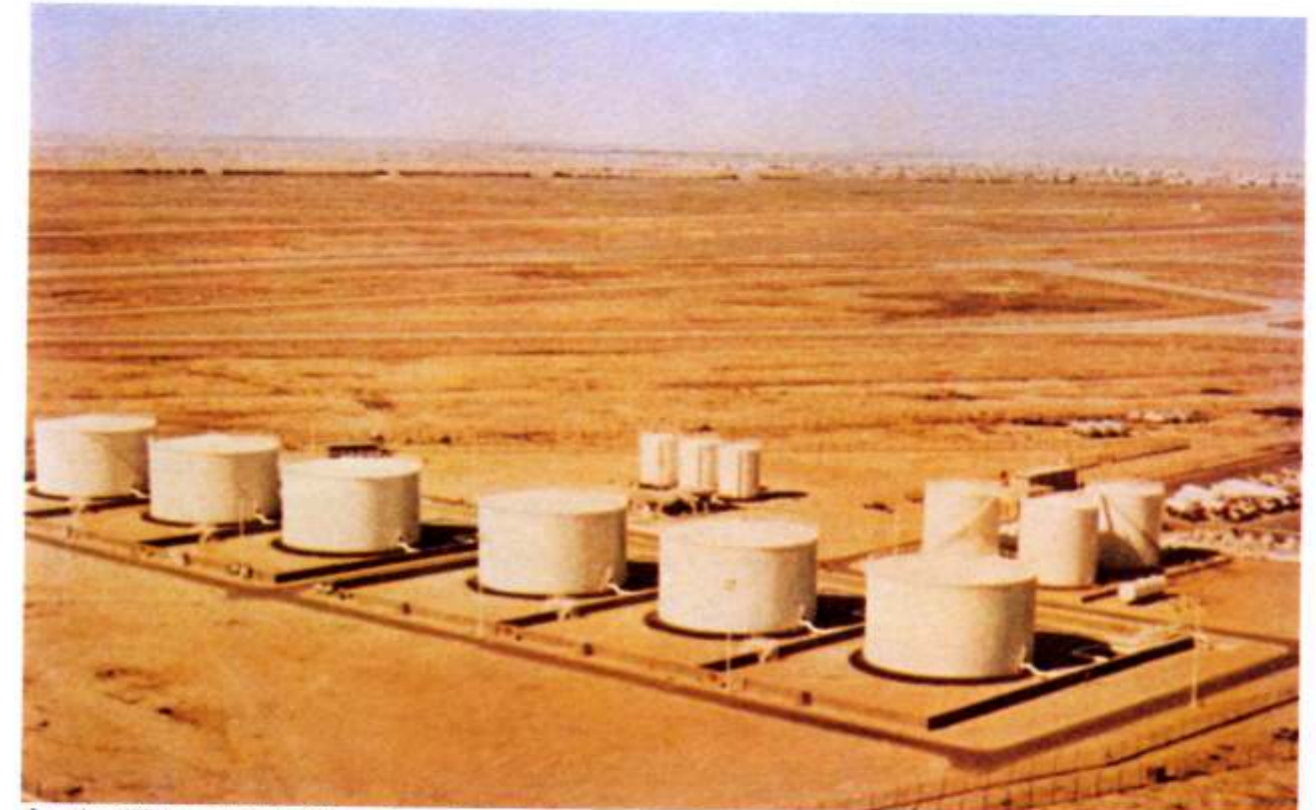
A turnkey ATF storage terminal designed, constructed and commissioned for KAFPCO, Kuwait. VTV's wide international exposure gives it an edge in terms of perspective in the implementation of quality systems.
