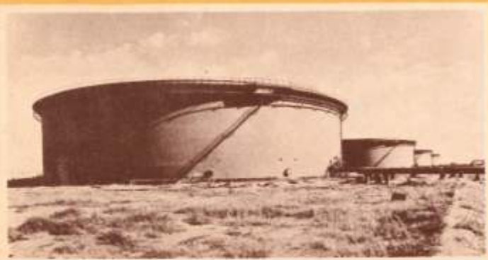
A View of a Crude Oil Storage Terminal at Vadinar where 8 x 90,000 M 3 tanks were constructed
