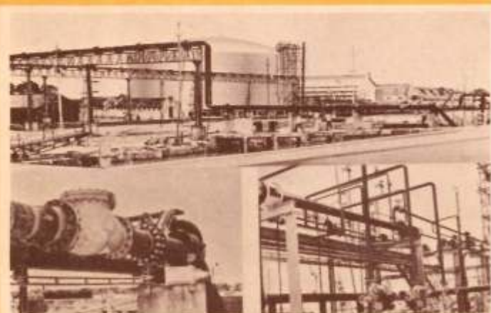
10,000 tonne double integrity ammonia tank with unloading facilities
