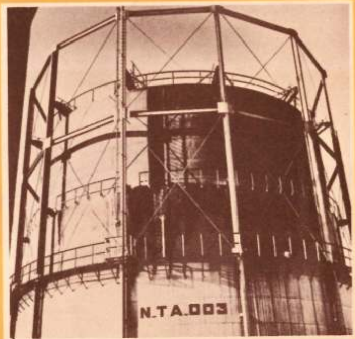
Double lift gasholder for Plastic Resins & Chemicals
