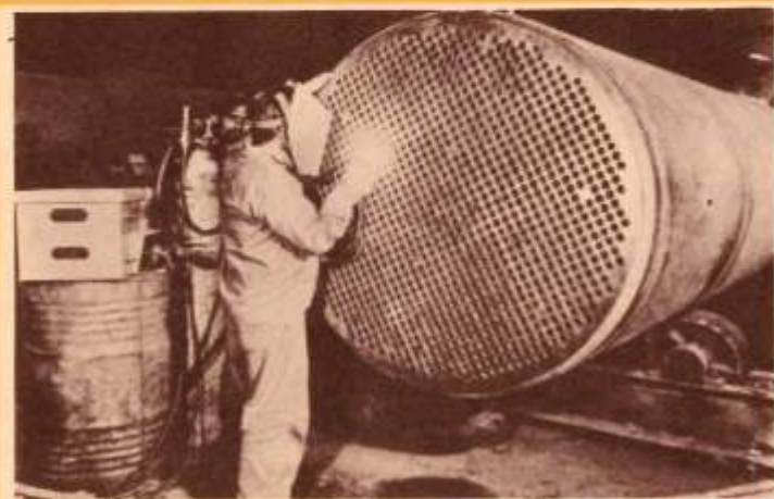
Stainless steel ammonia condenser under fabrication for heavy water project
