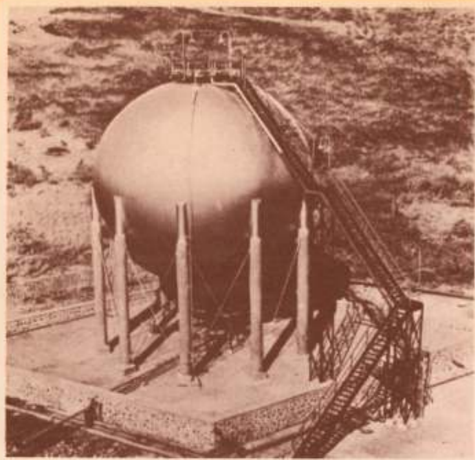
1,350 m 3 high pressure LPG storage sphere at Hindustan Petroleum Corporation
