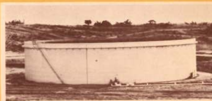
320,000 barrel crude oil floating roof tank
