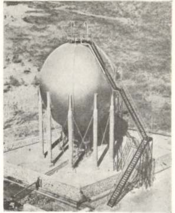
1350 M 3 High Pressure LPG Storage Sphere
