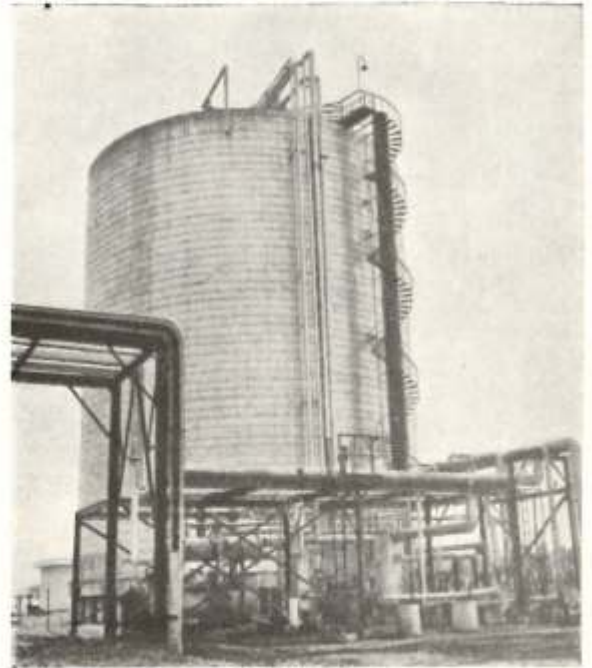
5000 MT Liquid Ammonia Storage Tank
